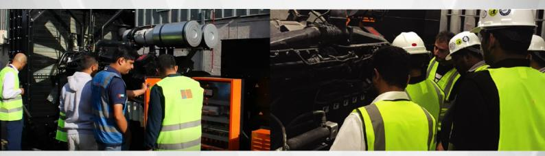
During the commissioning process, our team will simulate a power failure and test the generator's ability to engage and deliver the required power. This on-site load testing is crucial in verifying the functionality and performance of the generator.
