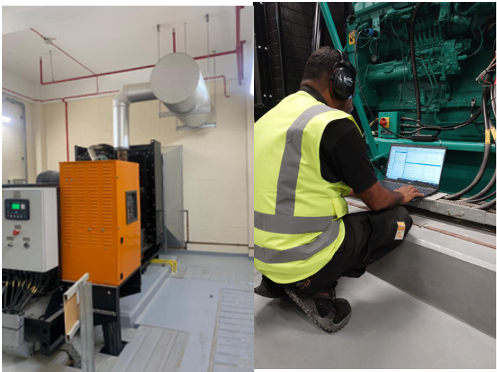
Electrical works and Controller installation with programming for more information page 8
