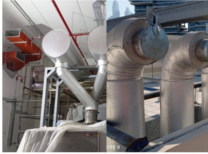
Generator Installation and fabrication works for more information page 3
